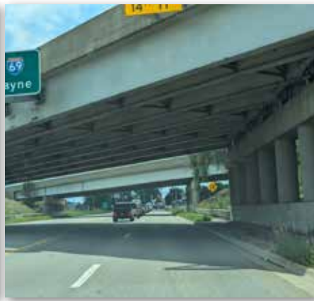
Lansing Rd I-69 underpass
