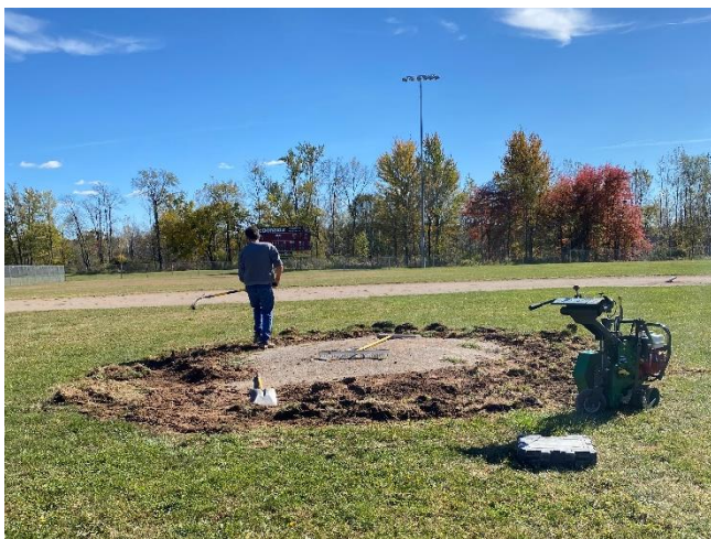
*Cutting out the lip, where the dirt and grass meets.
