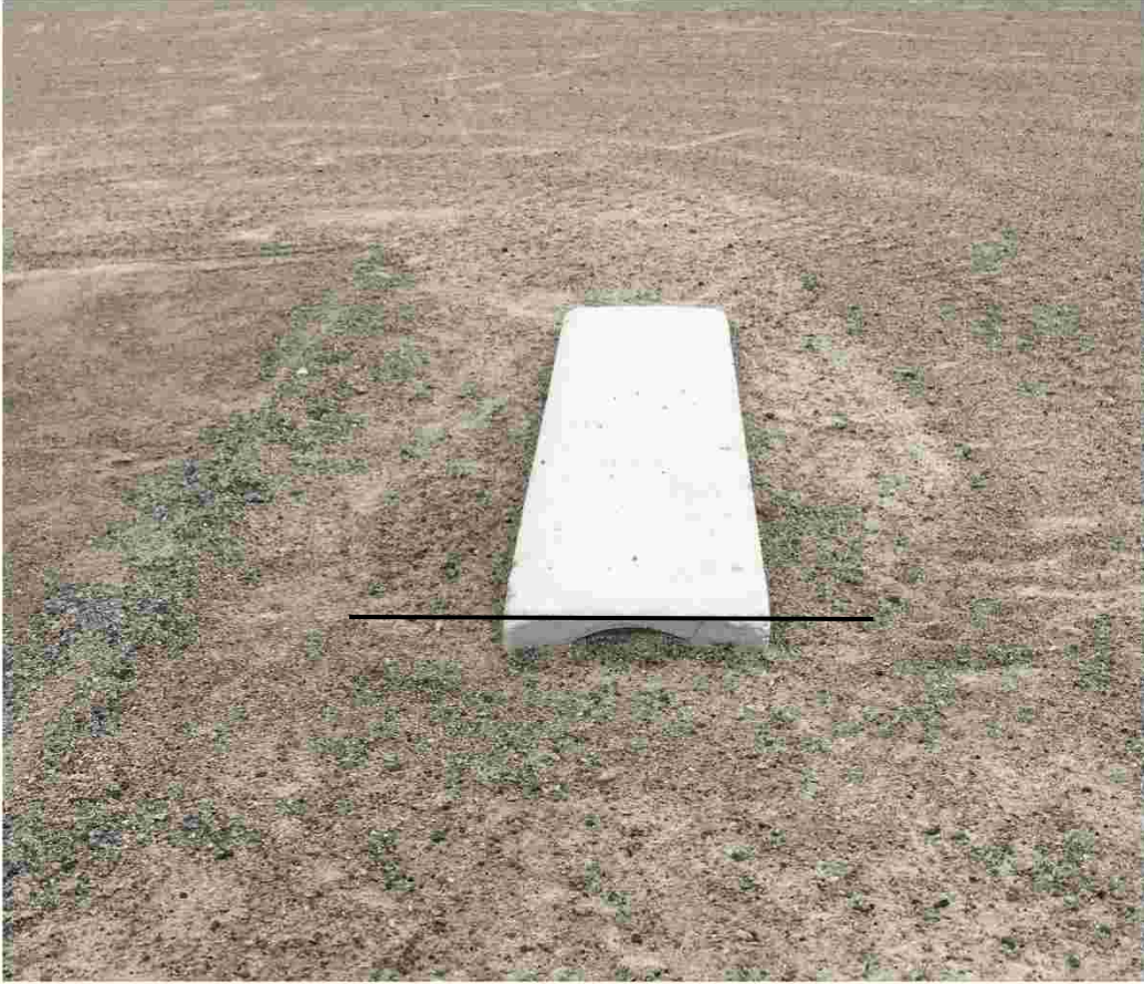
Pitching Rubber: dirt should be at the top part of the rubber- see black line
