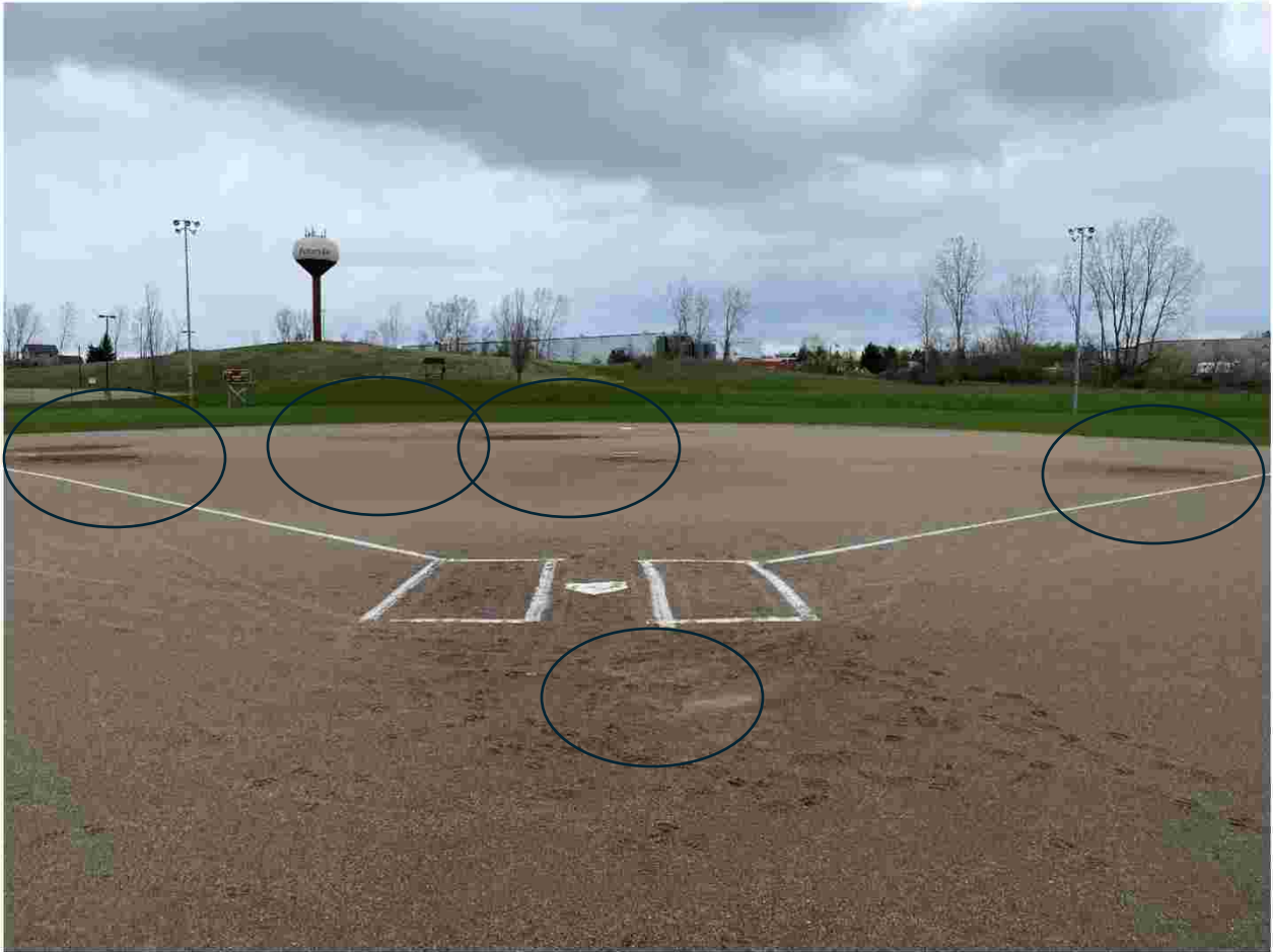
Multiple areas on each field with low spots.
