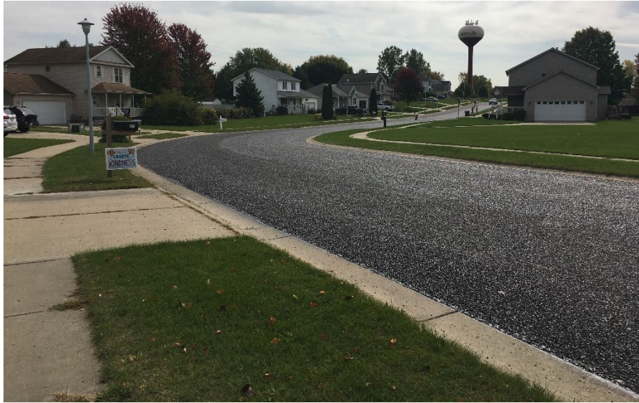
Figure 6: Road with Chip Seal and Fog Seal
