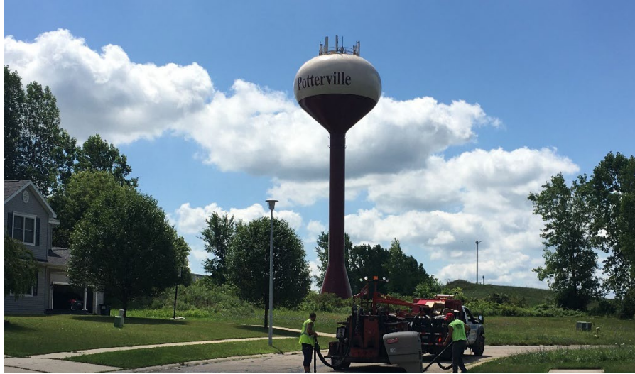
Figure 3: 300,000 Gallon Elevated Storage Tank
