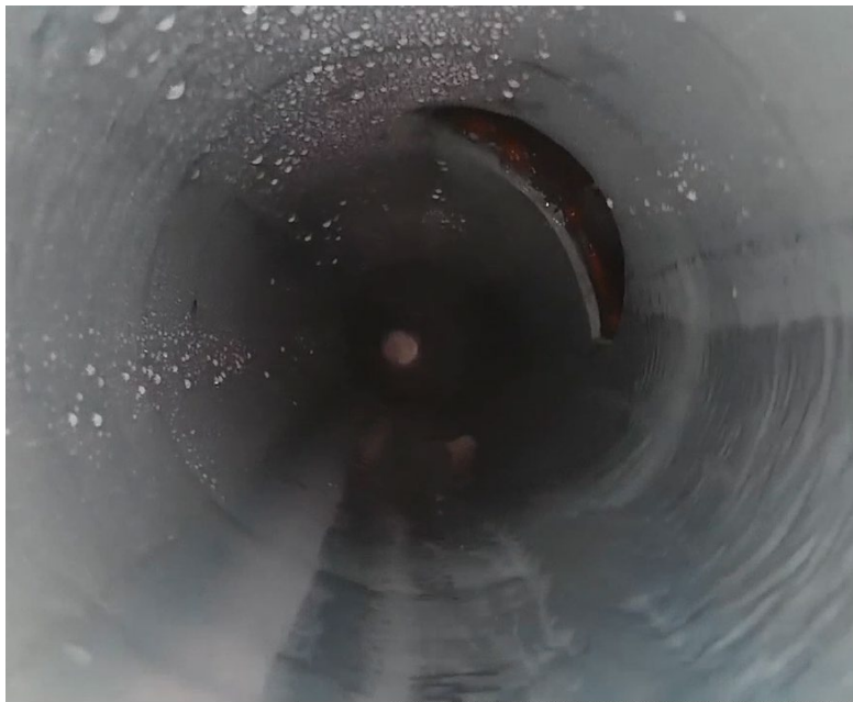
Figure 5: CIPP Lined Sewer with Lateral
